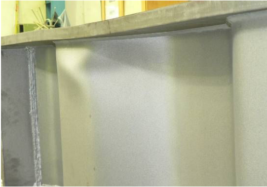
Figure 45: Failure mode of test specimen #10.
